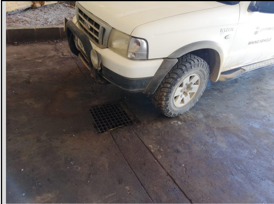
Picture 4: Wash bay
