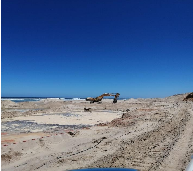
Ramp 3 - 5M buffer observed
